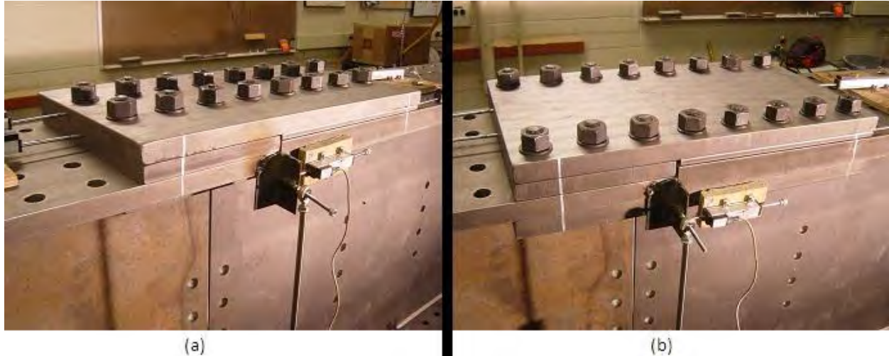
Figure 21: Filler 1 in Thick utilizing (a) inner flange holes and (b) outer flange holes.
