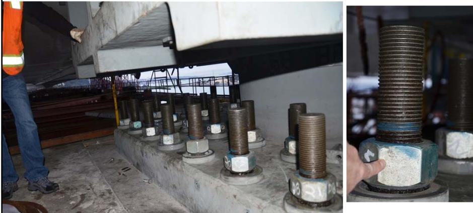
**32 of the 96 (2008) A354 BD anchor rods on shear keys S1 /S2 on Pier E2 failed after being tightened to specified tension levels**
